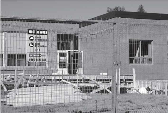
Photo: Espanola High School renovations will continue through the summer.
